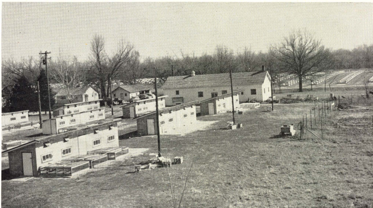
This view shows many of the buildings of the Pittsburg quail hatchery. The brooder houses are in the foreground and the holding pens in the background.
